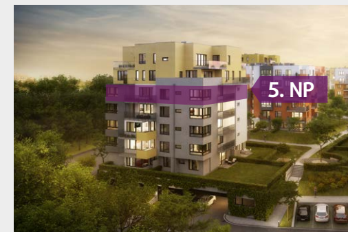
Pohled na dům / Building View
