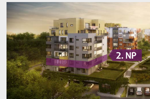
Pohled na dům / Building View
